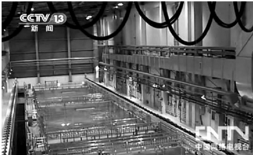
Figure 7. A cooling pond at China's pilot reprocessing plant. The plant has the capacity of processing 50–60 tons of spent fuel per year and began operating in 2011. The hot testing of the plant in 2010
